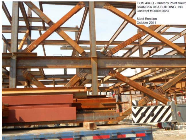
Figure 17: Lateral bracing erected
