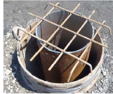
Figure 9: Isolation Casing Photo by SKANSKA Inc.
