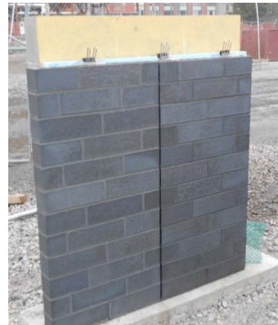
Figure 4: Typical Wall mock-up Photo by SKANSKA Inc.
