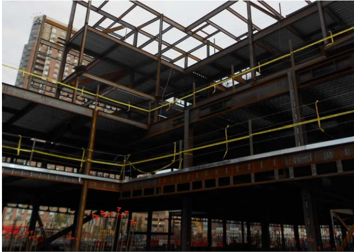
Figure 14: Steel Frame Erection Photo by SKANSKA Inc.
